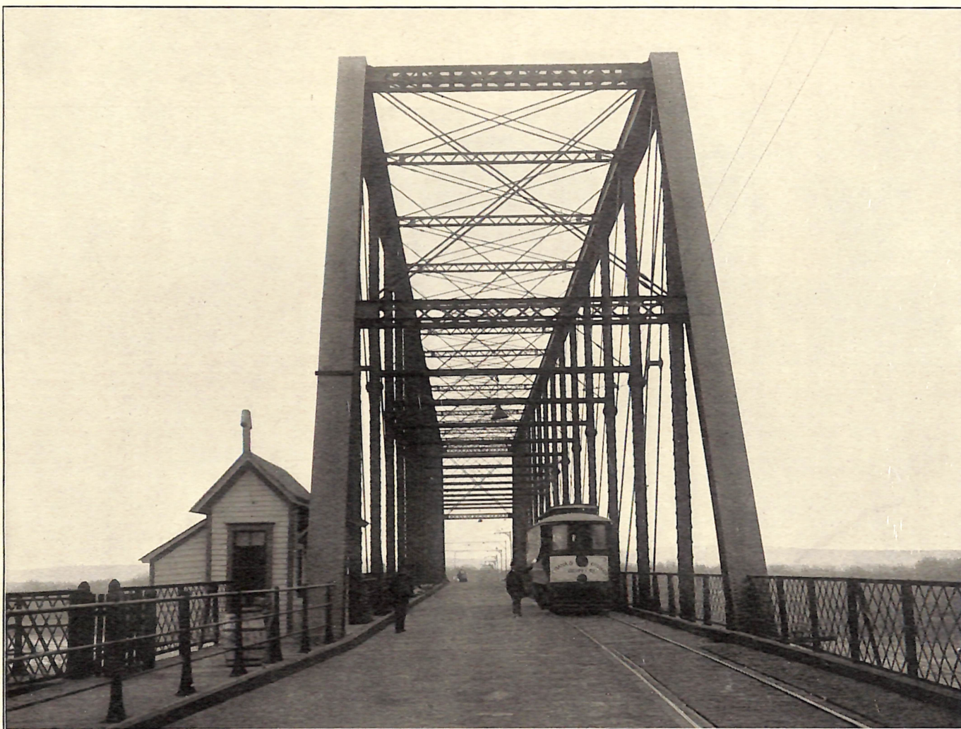
MIDDLE SPAN OF MISSOURI RIVER BRIDGE, O. & C. B. RY. & B. CO.
