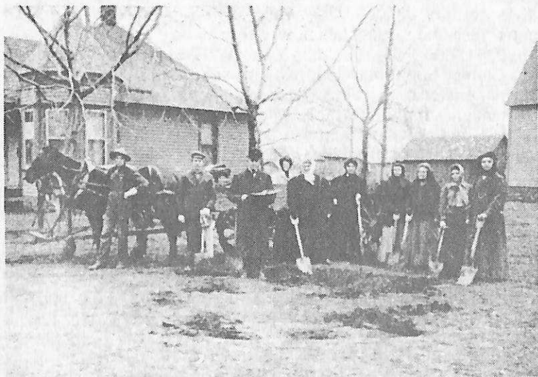
Ground breaking 1909. Epworth Methodist Episcopal Church.
